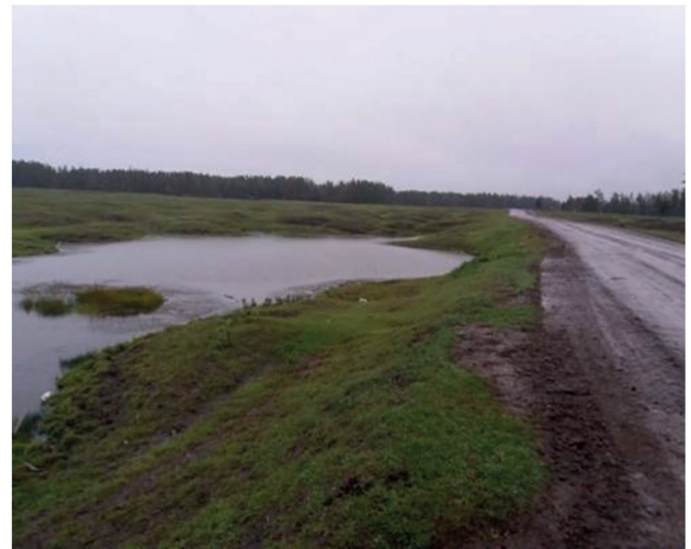
Fig. 1. (a, b). A typical remote sensing image of emerged thermokarst depressions along a road: a) high-resolution remote sensing data, GeoEye image b) photo
