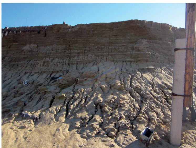
**Fig. 2. Sheet erosion of the techno-eluvium surface**
