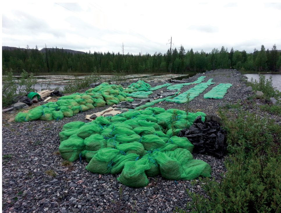
Fig. 2. The plastic mesh bags consist of sawdust, thermovermiculite, and seeds mixture
