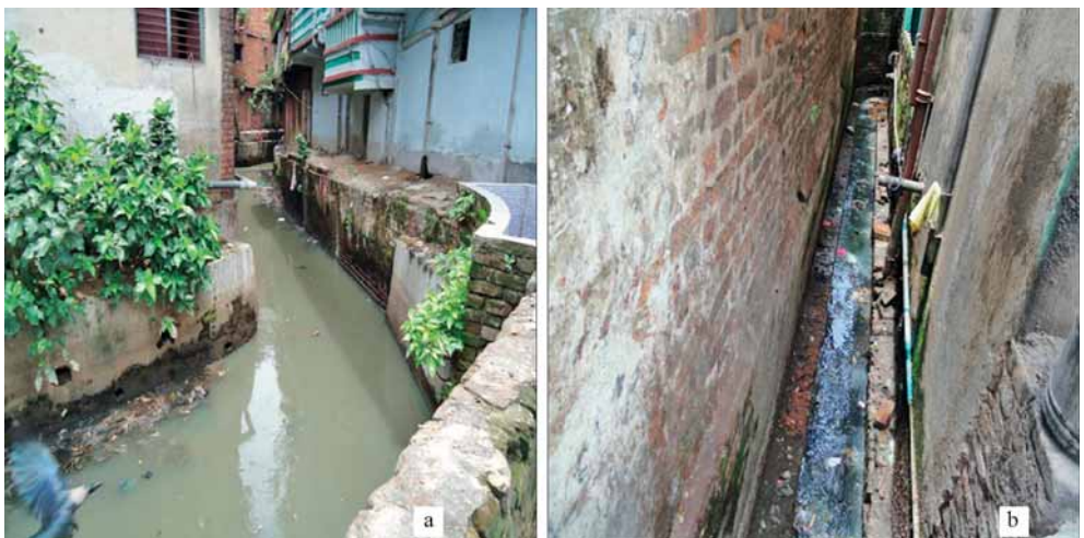
Fig. 4. Open drainage in Garden Reach, Kolkata.
