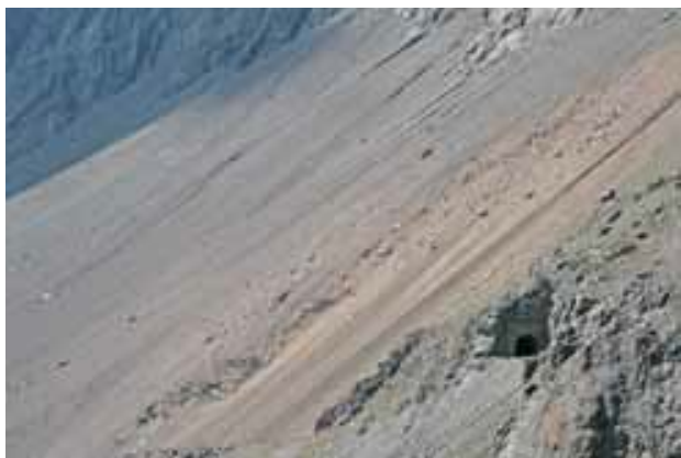
Fig. 5. Rockslides in the area of Cristo Redentor (Chile-Argentina border). The right low angle indicates the road tunnel entrance
