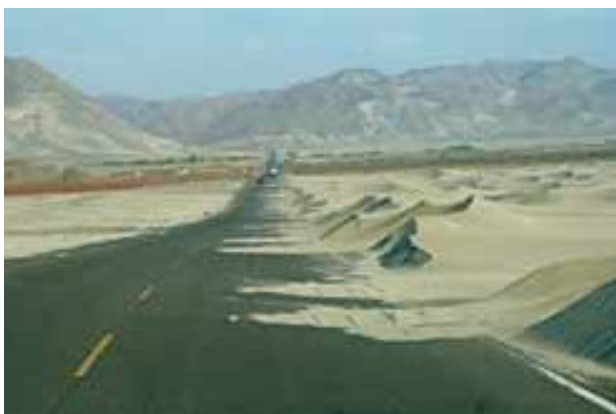
Fig. 7. Permanently moving eolian sands choke up Pan American Highway (north of Peru)
