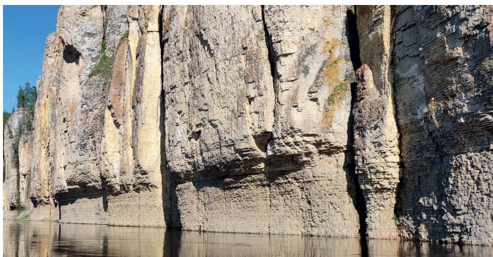
Fig. 5. Lateral river erosion expressed as niches on the base of limestone wall (at the «young ridge» site)
