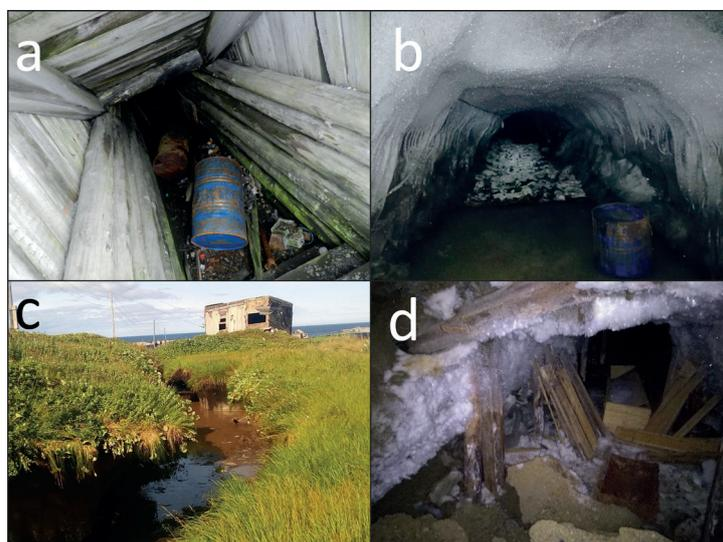
**Fig. 6. Primary issues with ice cellars in Chukotka: a) flooded cellar in Uelen (August 2014); b) molds on meat in the Inchoon cellar (August 2017); c) ice wedge thaw near the cellar in Inchoon (September 2019); d) sloughing walls and rock fall in the Lorino cellar (September 2018). Photos by A. Maslakov.**
