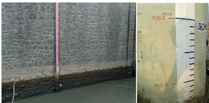
Fig. 1. Manual water level monitoring on river Jhelum
