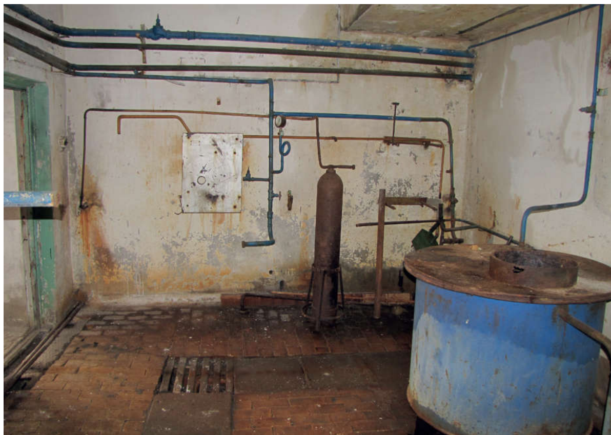
Fig. 2. Dysfunctional chlorination chamber, Sharyngol WWTTP
